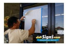
Hold the masking an inch from the glass at an angle.
