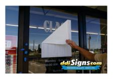
Slowly pull the masking off leaving the etched decal on the glass.
