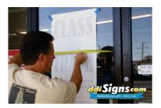
Line up the decal. Tape the corners to hold in place.
