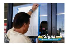
We use a side hinge of tape to hold the section in place. If left handed Hinge on left side.
