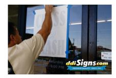
Run the squeegee over the masking to make sure the decal is adhered to the masking.
